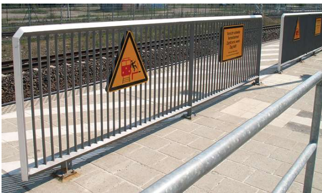
Fig. 4.10: Barricade for queues and access control
